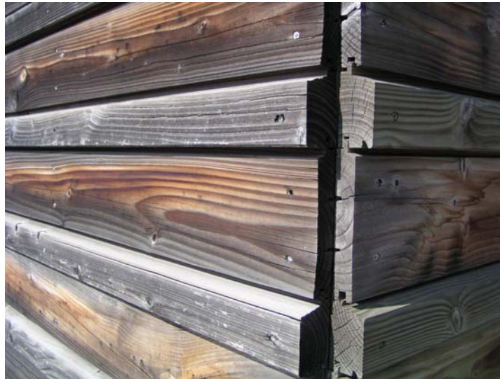
Figure 5: Influence of the cladding profile on wood greying
