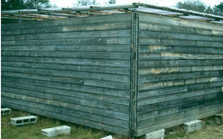
Figure 1: Scots pine cladding, sides facing west (on the left) and south (on the right)
