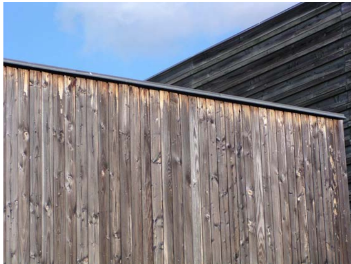
Figure 4 : Influence of the design on wood greying
