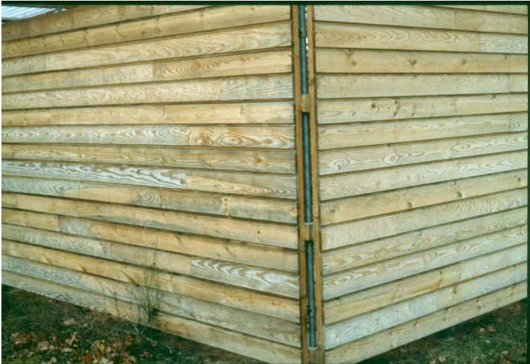
Figure 2: Scots pine cladding, sides facing north (on the left) and east (on the right)
