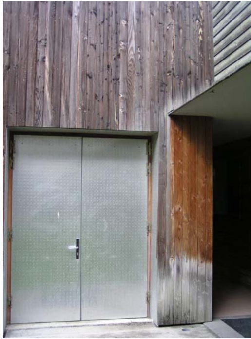
Figure 3 : Influence of the design on wood greying
